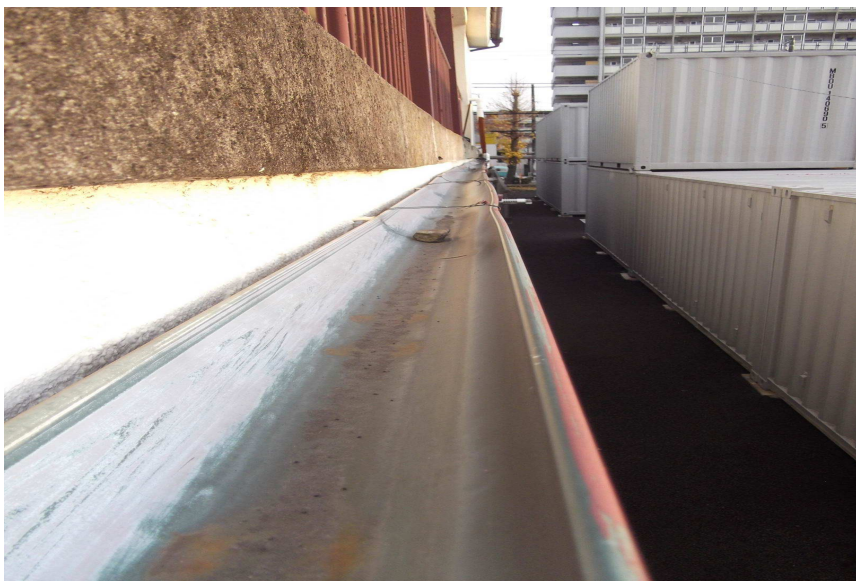
1F軒樋歪み・破損
